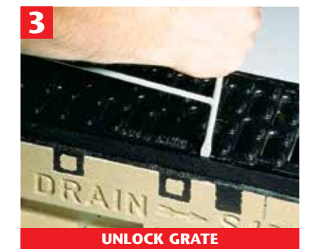
3 UNLOCK GRATE Rotate tool 90°; PowerLok device should push away from rail.
