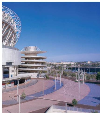
Main entrance to Stadium Australia, note curved runs of S170 drain were used at change of brick paver colour
