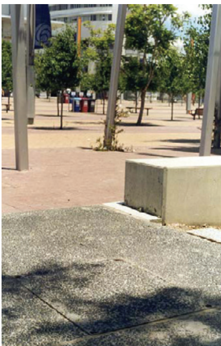
Recessed galvanised steel ACO access cover filled with concrete located in the Public Domain next to the Overflow area
