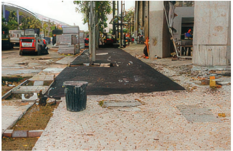
ACO access covers being installed in brick paved area alongside the hotel. Olympic Park railway station can be seen in the background
