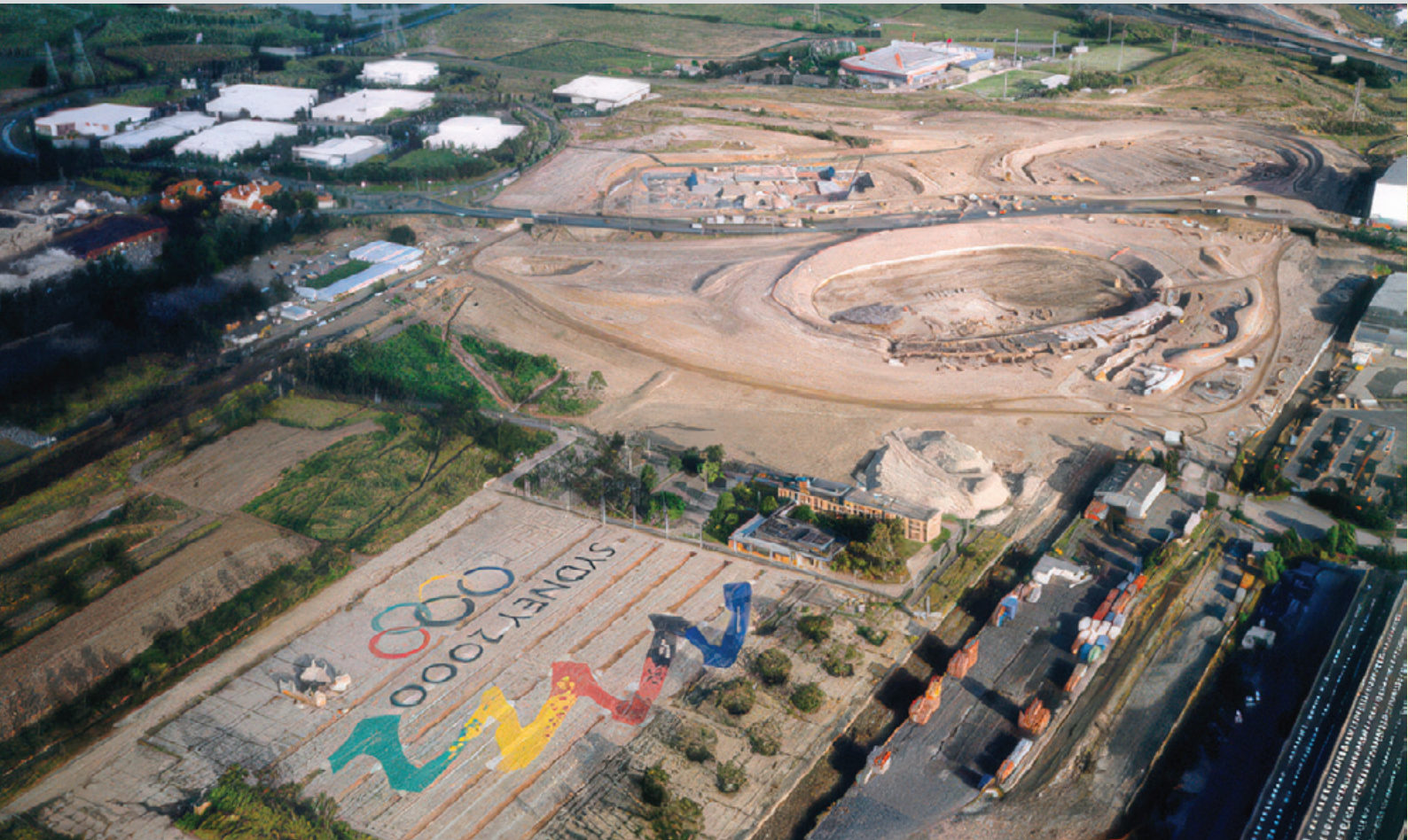
Aerial view of Homebush and the construction of SIAC
