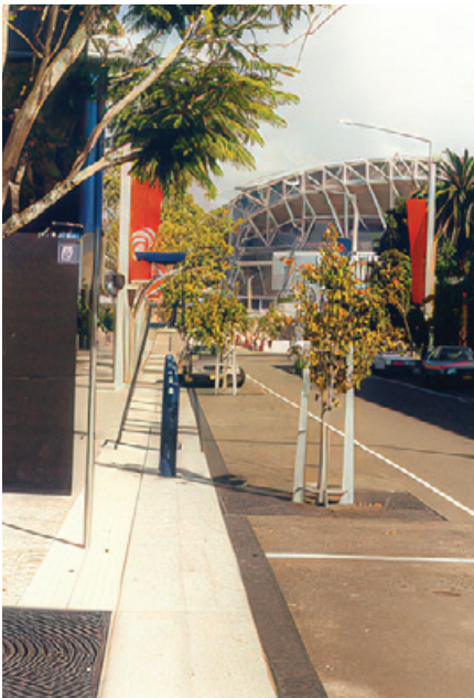
Completed S170 drain alongside Railway Station
