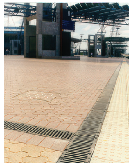
S170 used along the sides of Dawn Fraser Avenue to drain the Public Domain
