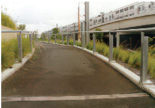
On the wheelchair ramp off Australia Avenue, ACO Drain K100S and Heelguard 'S' stainless steel gratings were used on the 6 runs
