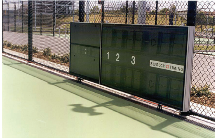
Rosette gratings and K100S in front of scoreboard on outside courts used for preliminary tournament matches
