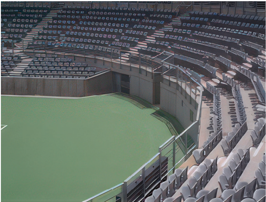
Centre Court - the K100S runs along the edge of the court and the rubber surface is laid over the gratings and the holes cleaned out afterwards
