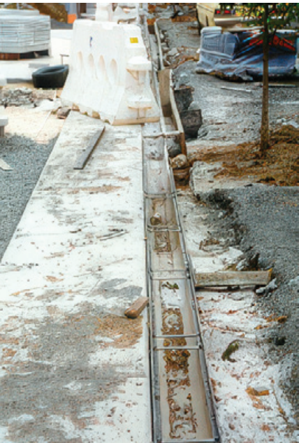
S170 drain being installed alongside the Railway Station
