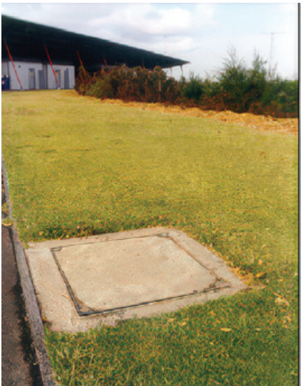
Brass edged ACO access covers were used on top of the polymer concrete electrical pits
