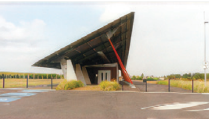
The unusual shaped roof of the Archery centre
