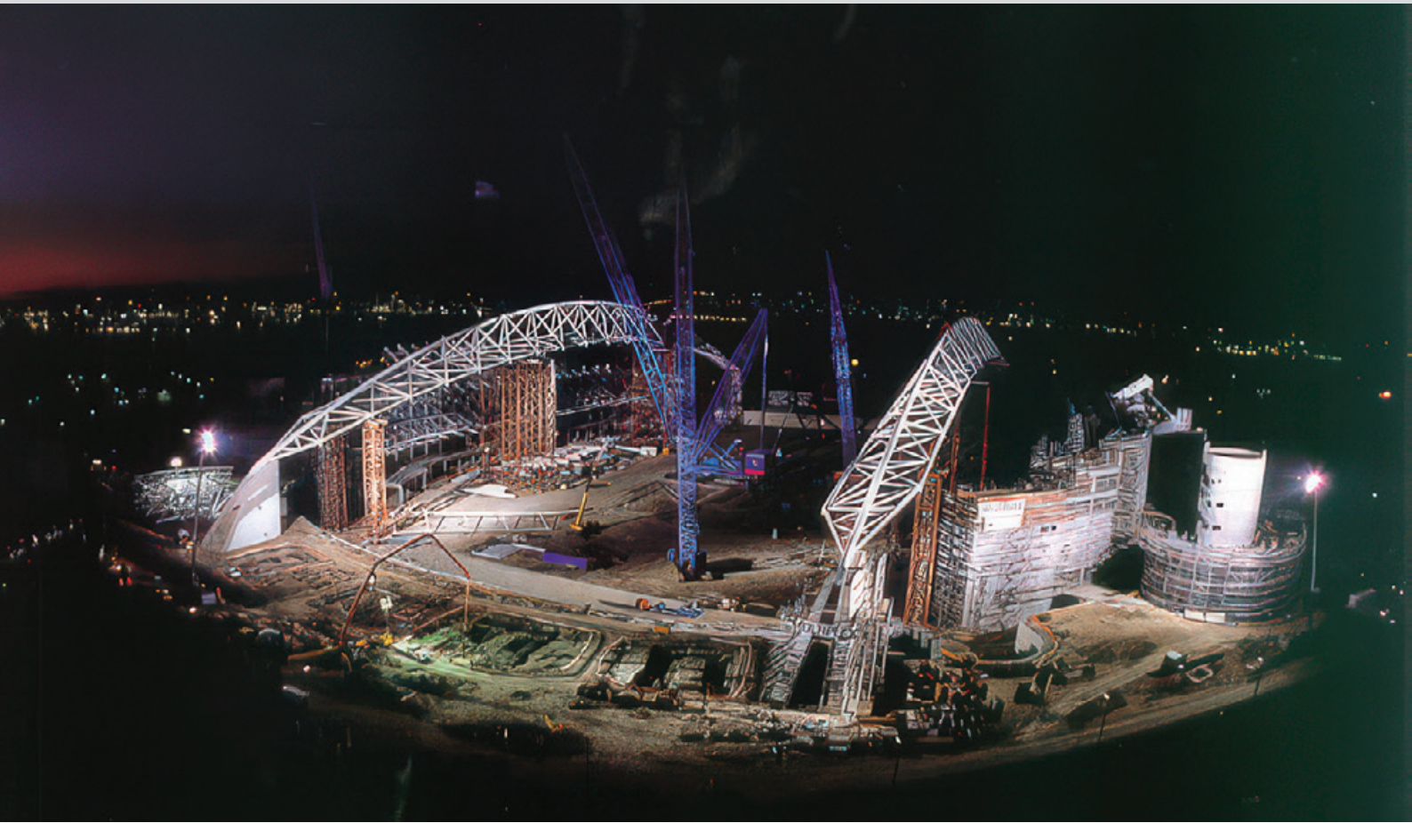
Stadium Australia under construction
