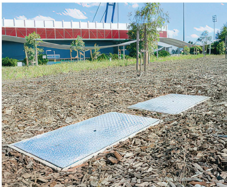
Solitary irrigation valves used either Type 52 or PEP 22 earth rod pits with galvanised steel chequer plate covers
