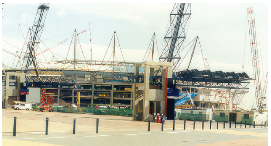
The Superdome under construction, note that the dome roof had not been erected
