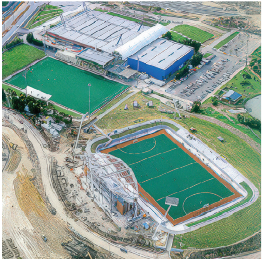
The Hockey Centre (top left) during construction, the pitch top left is the original international venue which will be the warm up pitch during the Olympics
