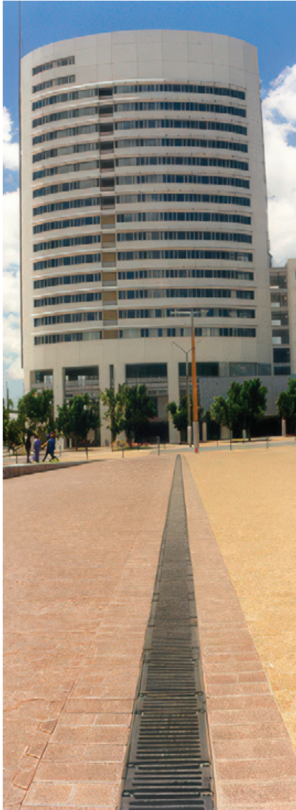
ACO Drain S170 from Fig Grove water feature to the Olympic Park Hotel
