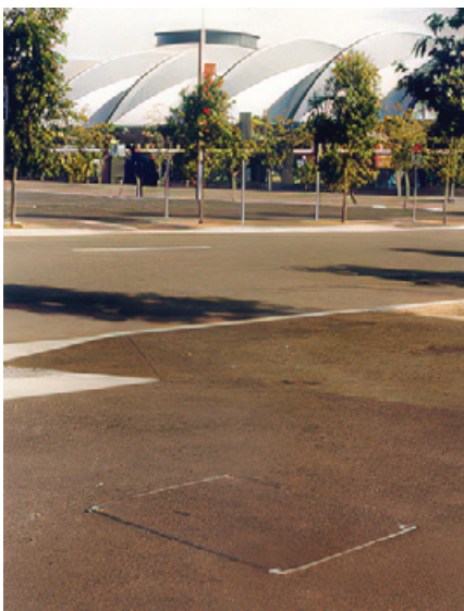
Recessed steel access cover above polymer concrete electrical pit in asphalt footpath
