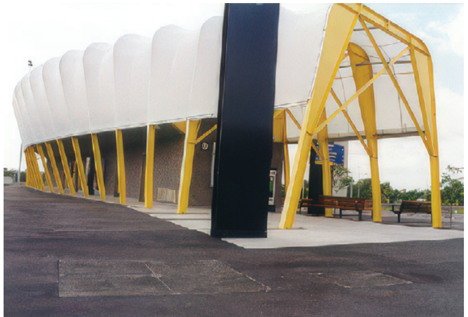
At various points around the site located by car parks or bus stops are amenity blocks. In front of the block is a single ACO access cover on an electrical pit and a four part unit covering the sewer pumping system
