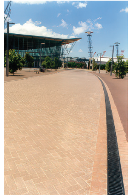
Curved runs of S170 in the area between the Superdome and the multi-storey car park, note the red-coloured bitumen areas either side of the brick paved roadway
