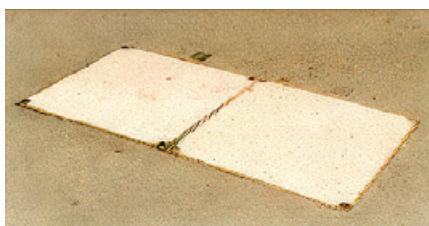
ACO access covers used in the footpaths around the animal pavilions
