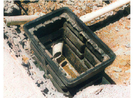
Type 5 electrical pit during installation on Overflow area in Public Domain
