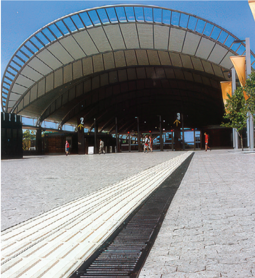
The S170 drain leading up to the Railway Station
