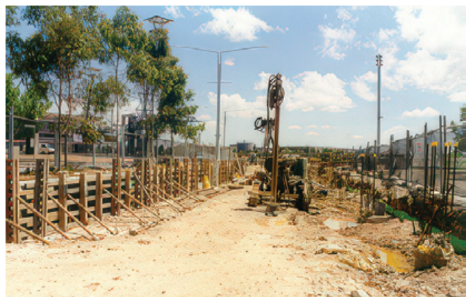
A late addition to the site was a bus underpass built at the bottom of Dawn Fraser Avenue, a further 200 metres of S170 was used here
