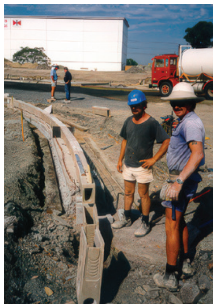
SIAC running track under construction and the polymer concrete drain system
