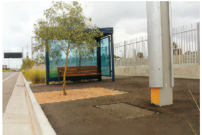
All light pole jointing boxes were supplied by ACO and covered with ACO access covers
