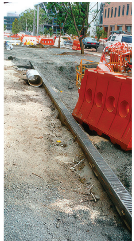
K100S and Heelguard grates during installation
