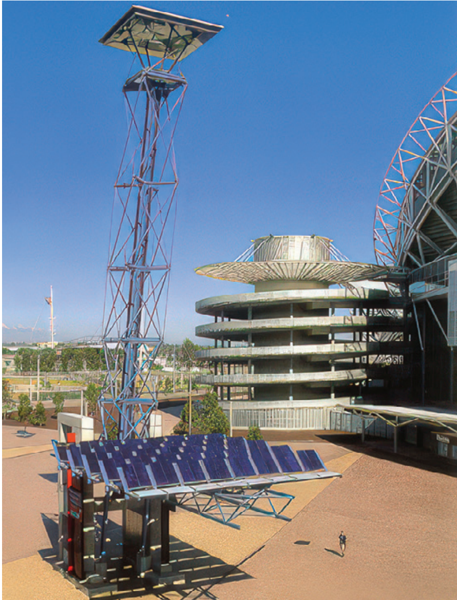
One of the light towers outside Stadium Australia, note the S170 in the foreground
