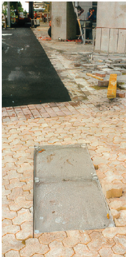
The two-part ACO access cover installed above the Type 8 electrical pit outside of the hotel
