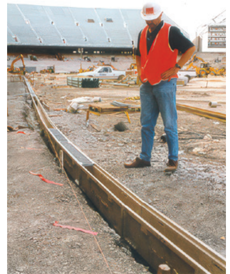
Main track drain during installation
