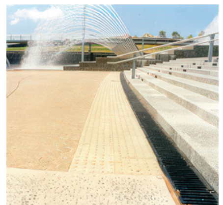
A run of ACO Drain S170 was located at the bottom of each of the three sets of steps at the Northern Water Feature
