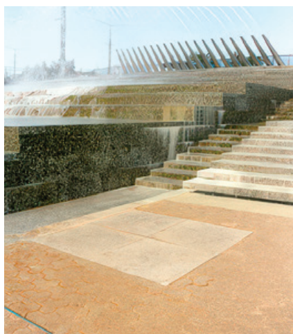
An ACO recessed galvanised steel multipart cover over the pumping system for the Northern Water Feature
