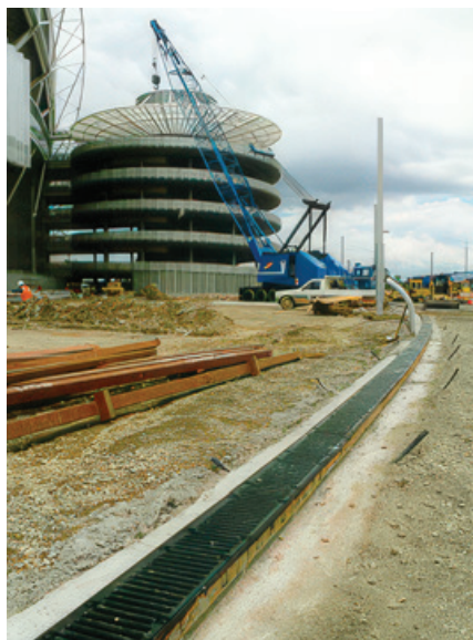
S170 being installed outside Stadium, note the curved run
