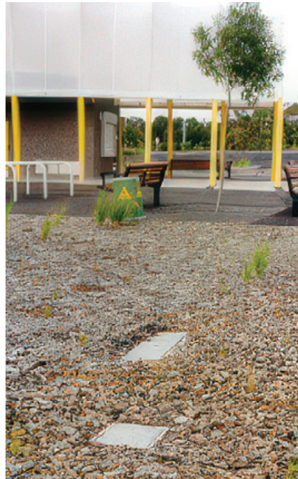
Solitary irrigation valves used either Type 52 or PEP 22 earth rod pits with galvanised steel chequer plate covers
