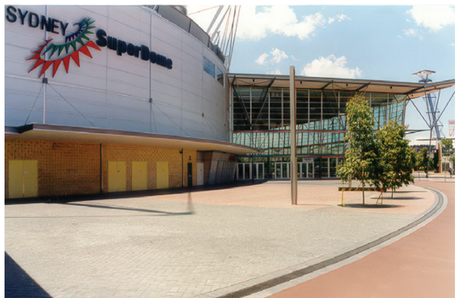
Curved run of S170 at rear of Superdome
