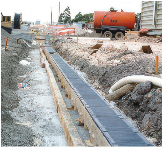
The first run of S170 channel on the Olympic site was on Australia Avenue
