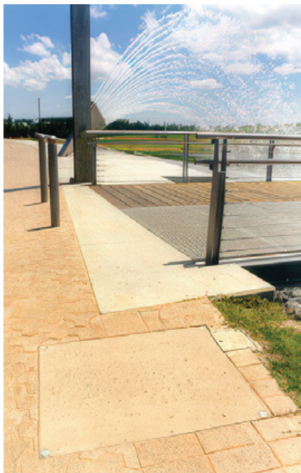
ACO 900 x 900mm access cover filled with brick coloured concrete, note the PEP22 earth rod box adjoining the cover on the right-hand side to cover a valve
