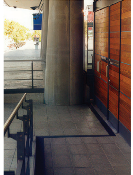
K100S with ductile iron Heelguard grates at doorway entrances to the station
