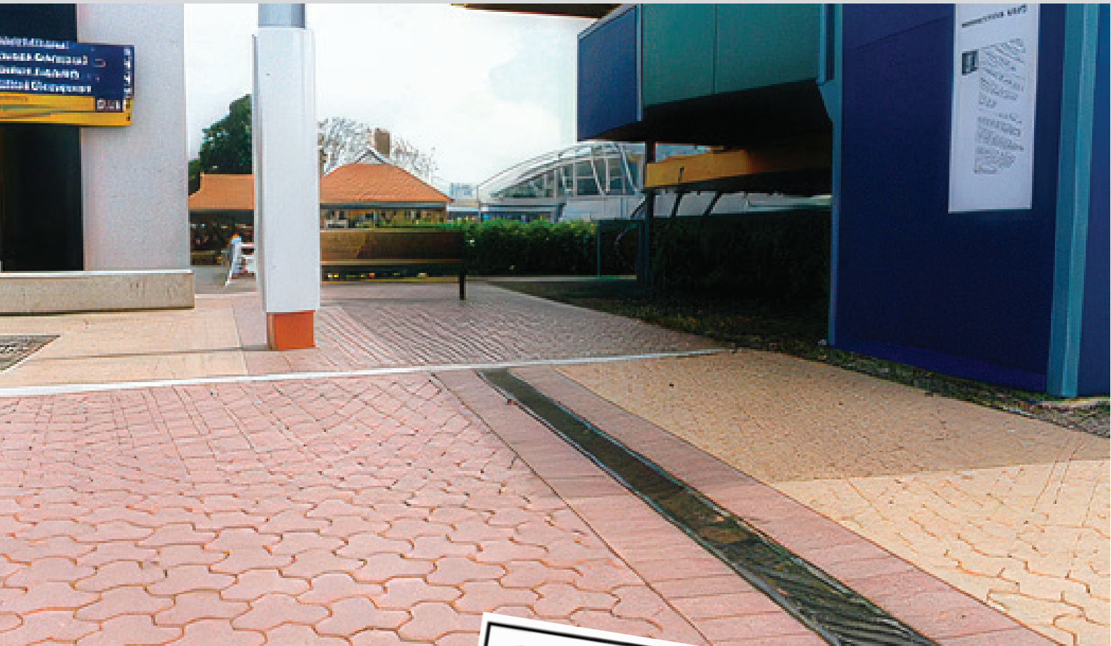
S170 installed in the test area
