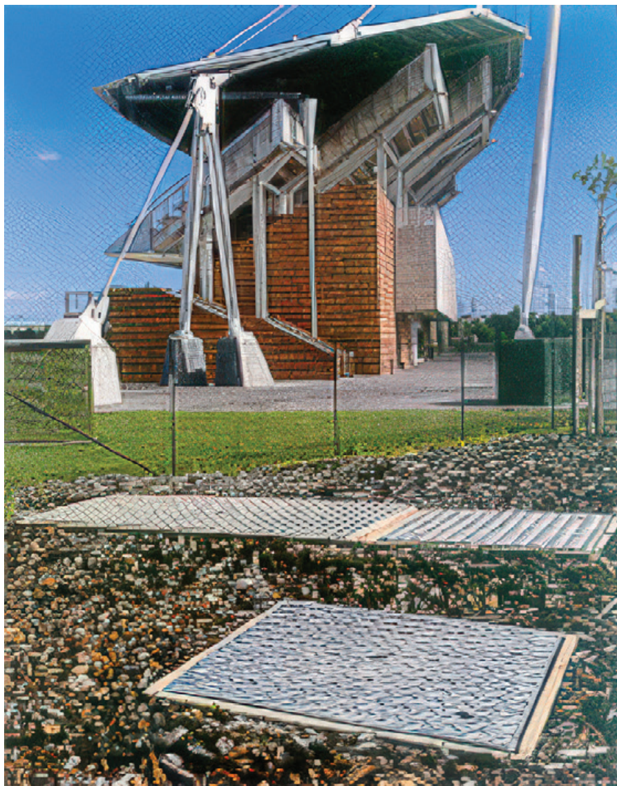
Polymer concrete pits and steel chequer plate covers outside the Hockey Centre
