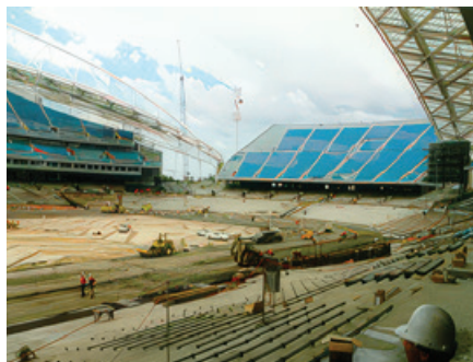
Stadium under construction
