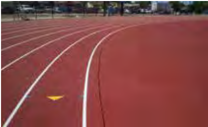
Straight & radius channels Radius channels to give a smooth line around curved areas of the running track
