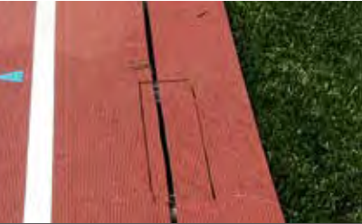
Drainage slot 13mm wheelchair compliant drainage slot offset from the centre of the channel
