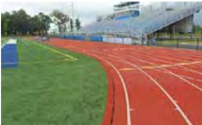
Straight & radius channels Radius channels to give a smooth line around curved areas of the running track
