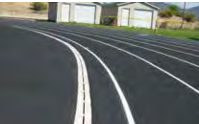
Polymer concrete surface Exposed edges will not rust or discolour surrounding surfaces
