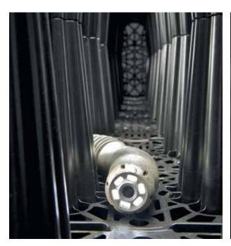
Inspection Cameras can be easily used in the ACO StormBrixx<sup>®</sup> system.
